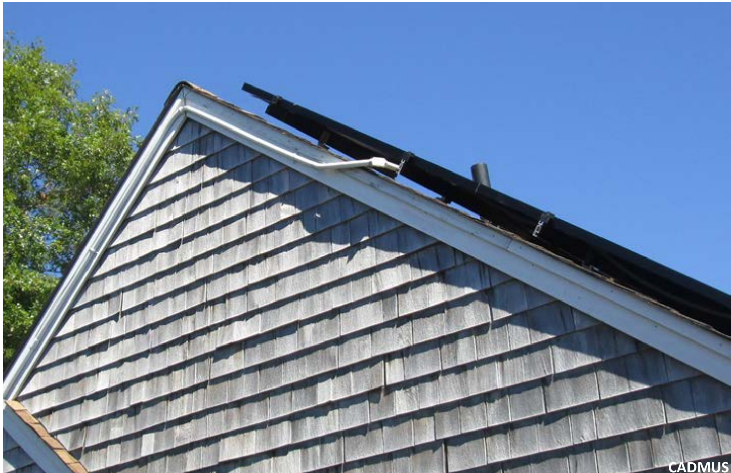
PV output conductors installed in conduit.
