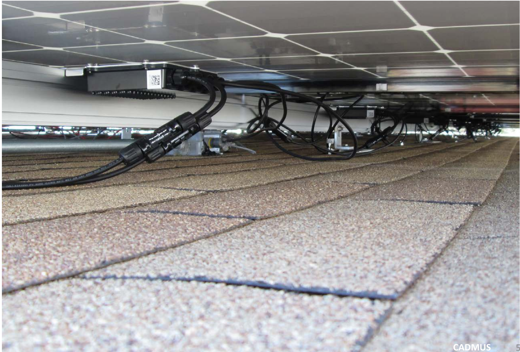
PV conductors are not supported under the array.
