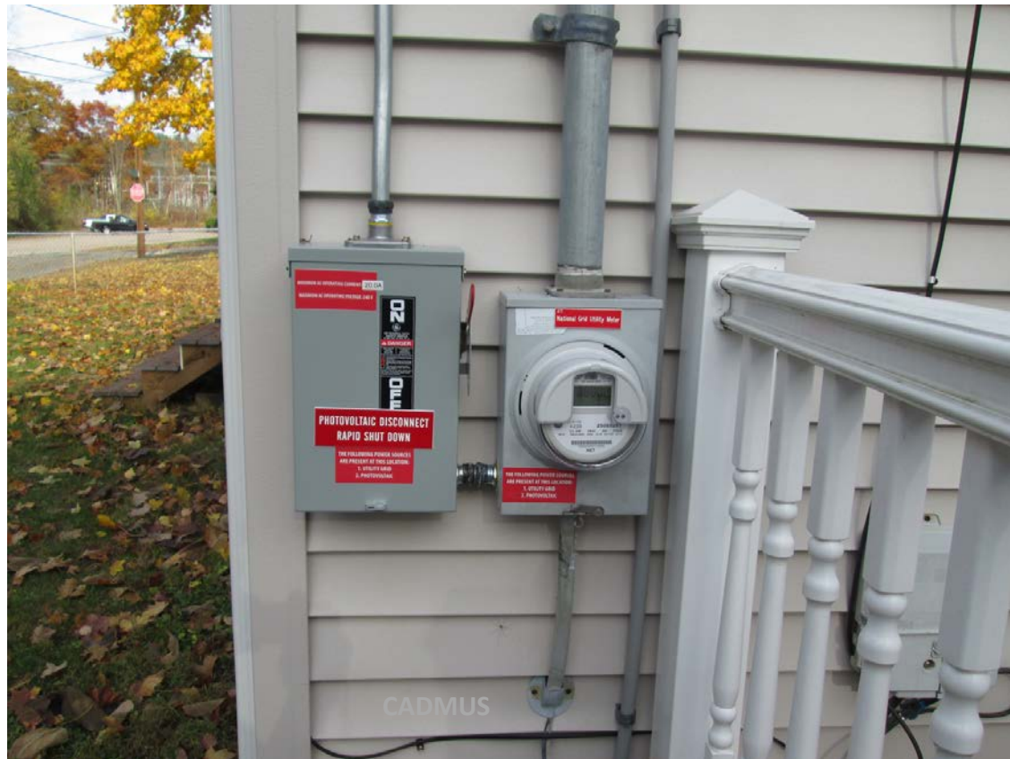
Connection is made inside the utility meter enclosure.
