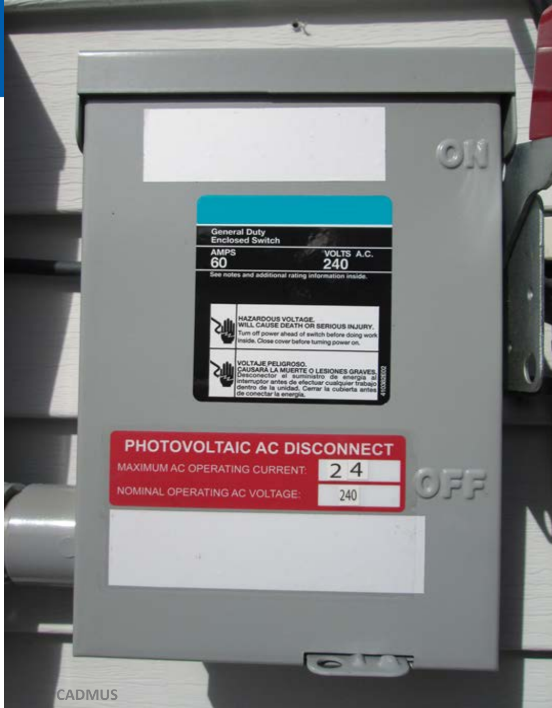
Labels are faded and not suitable for the environment.
