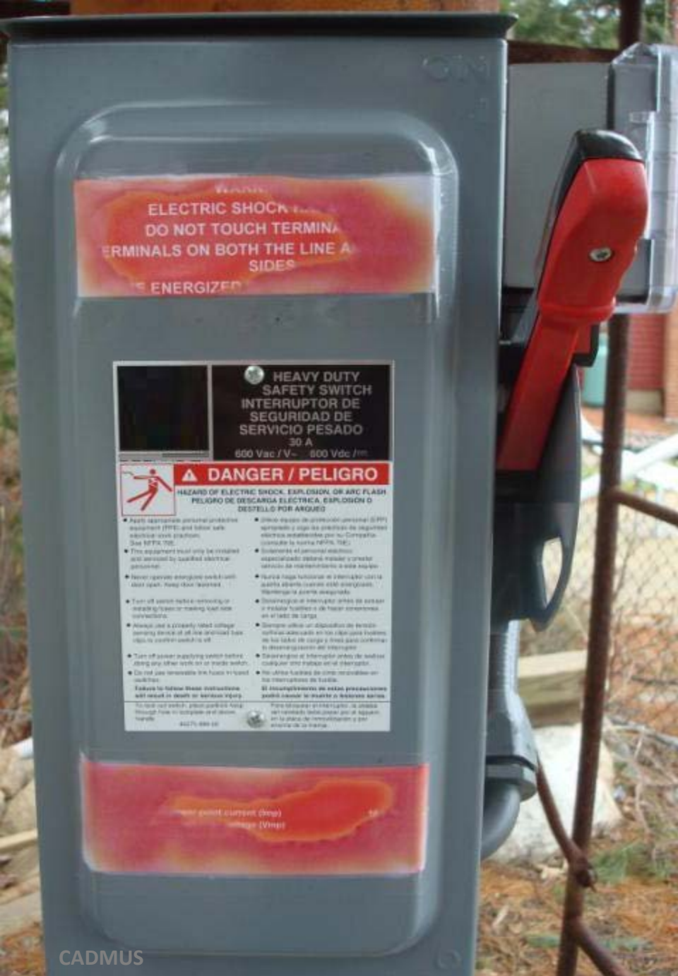
Labels are faded and not suitable for the environment.
