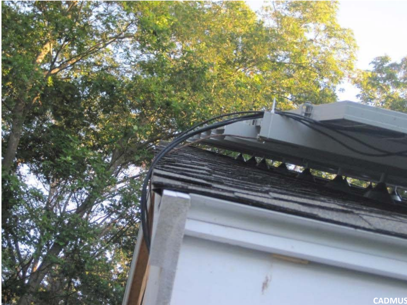
Unprotected PV output conductors.
