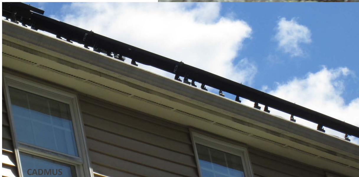
PV conductors are properly supported under the array. Upper photo taken from ladder, lower photo taken from ground.
