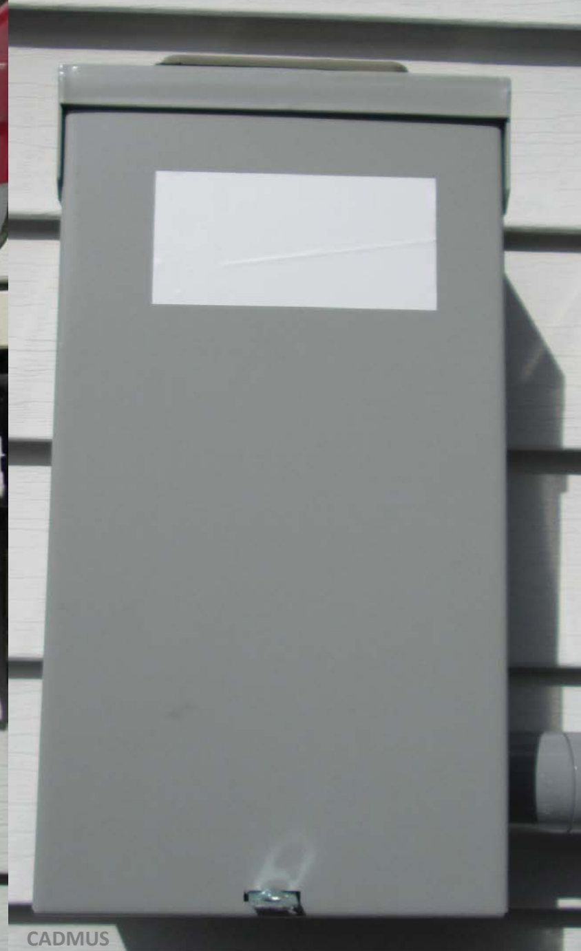
Labels are faded and not suitable for the environment.
