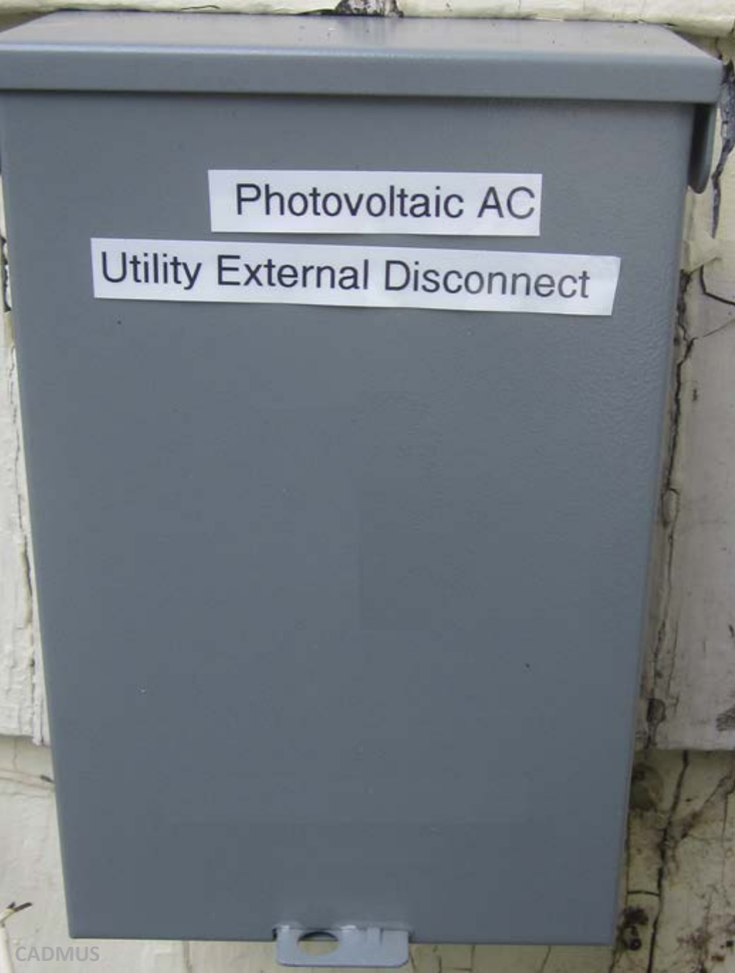
Labels are peeling and not suitable for the environment.
